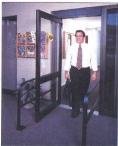
Automatic swinging doors are best suited for one-way traffic.
